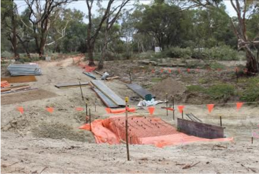
Photo 2: Preparation works has commenced at Katfish Reach.
