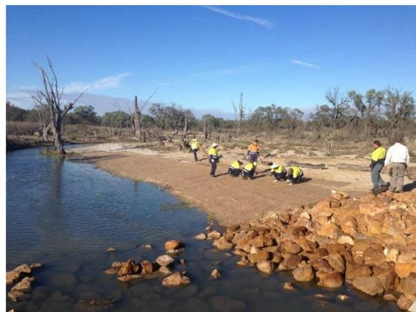
*Photo: Jute Mesh being installed by the Green Army with assistance from John Mitchell and Wayne Ahrens*
